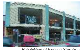
Rehabilitation of Existing Storefronts
