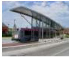
Bus Rapid Transit Station Cleveland, OH
